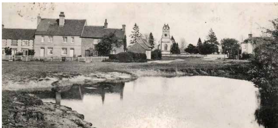
A view of the cottages and the church from the green
